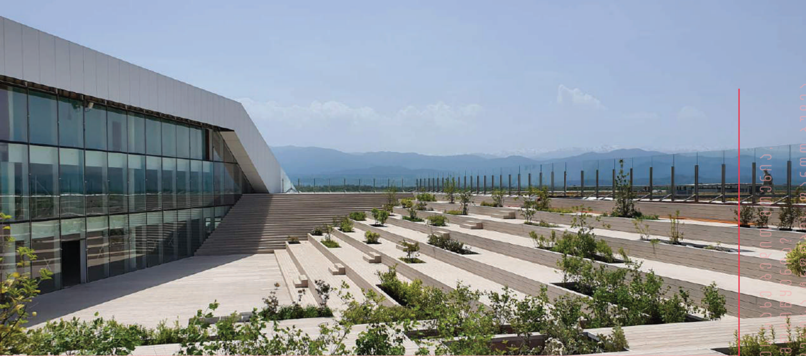
33 The green roof on the airport's second floor
